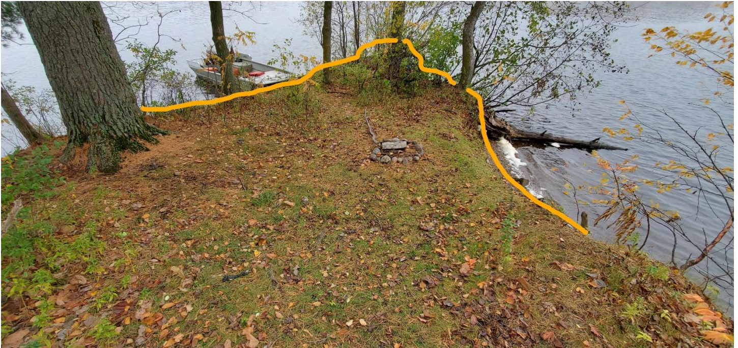
This is a view of the west end. The rock will extend around the tip.
