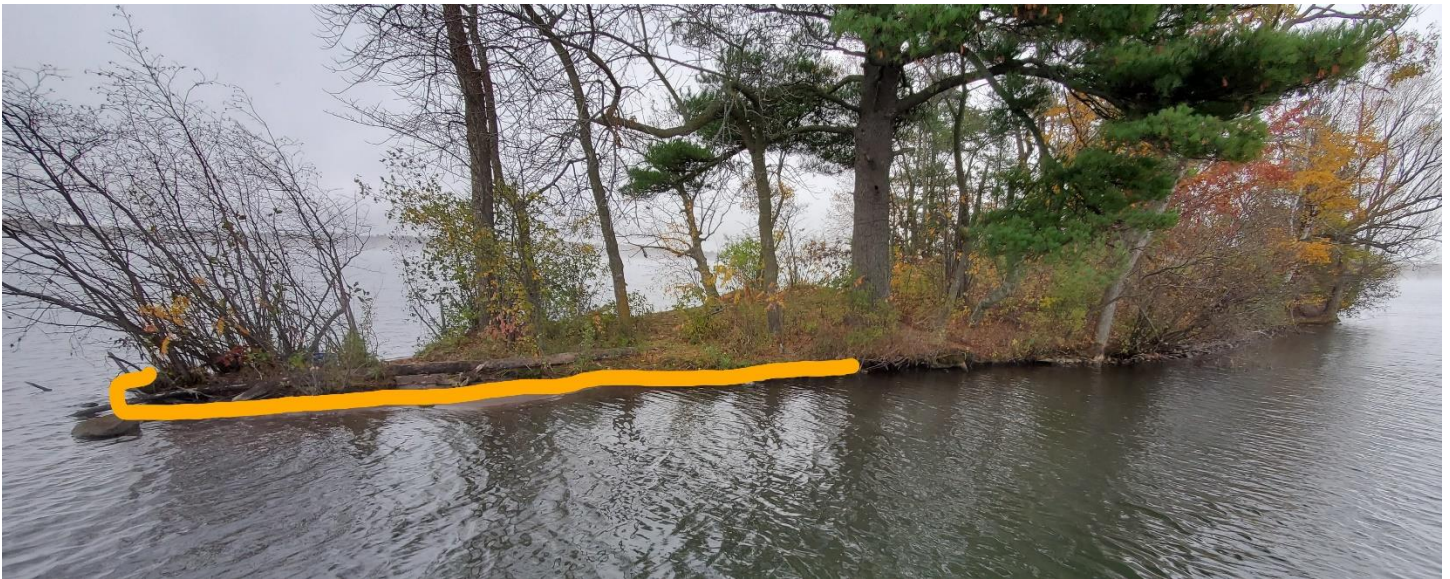
On the west end of the island the riprap will extend from the large white pine around the tip.
